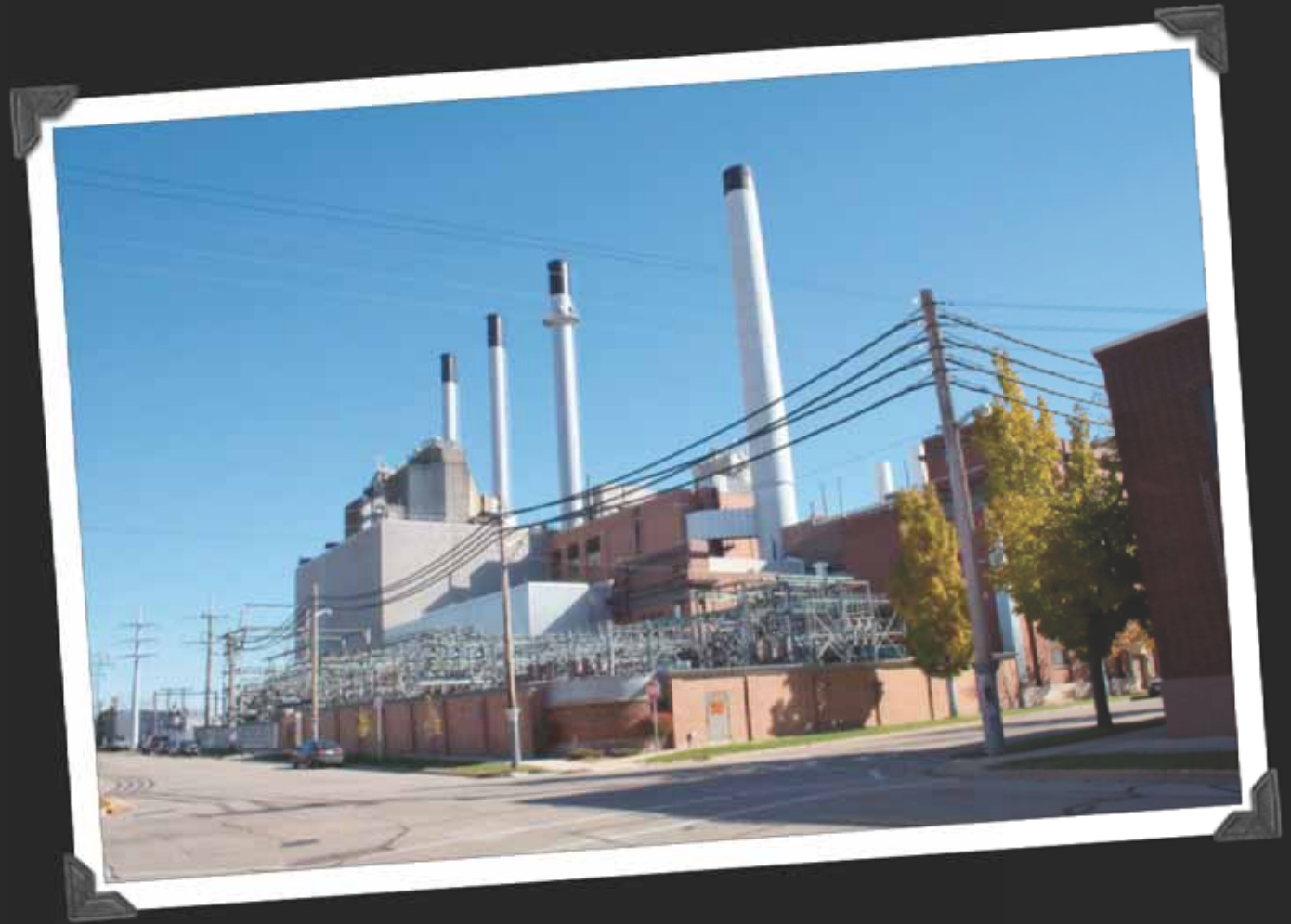
Madison Gas and Electric Blount Street Station
